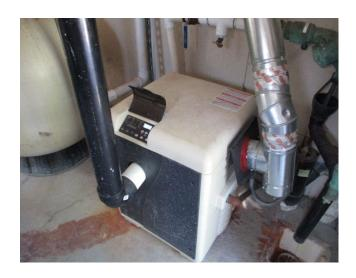
These are the pentair master temp 400 pool heaters located at the belltower pool:
