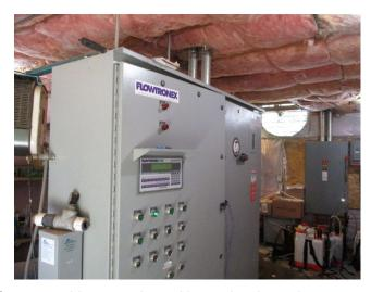
This is the Flowtronex variable frequency drive control panel located at the main pump station.
