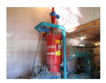
This is the irrigation filters located at the main pump house and ustick pump house:
